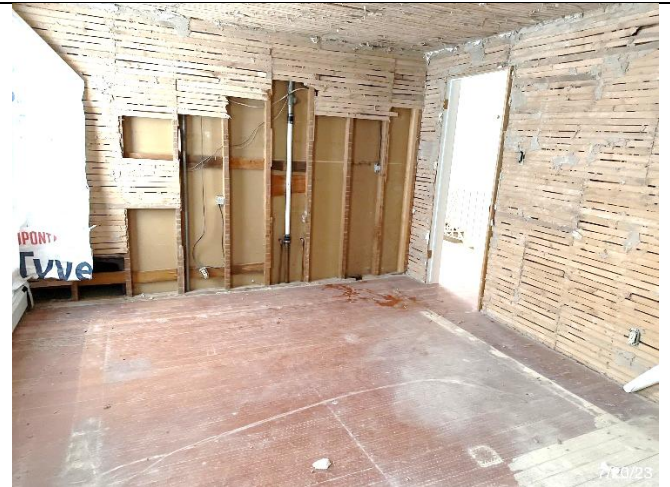
Bedroom 3 upstairs with the culprit revealed and repaired.
