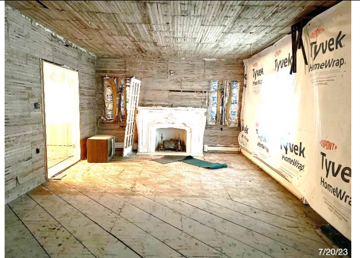
The fireplace end – showing walls, floor, and ceiling stripped down to the original bare wood.
