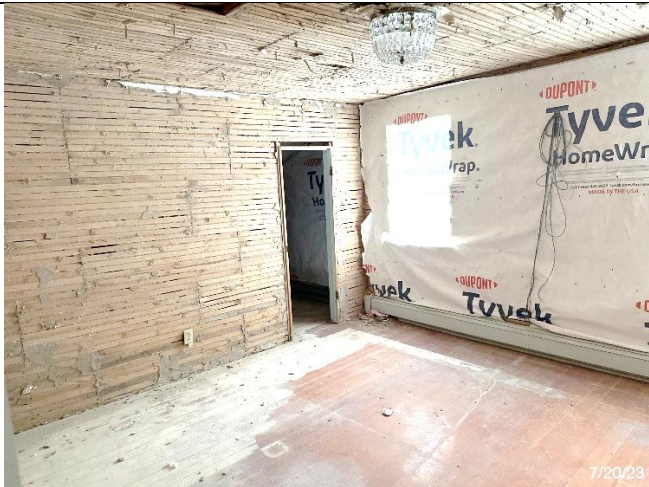
Upper-level Bedroom 3 – remediated and showing the original lath
